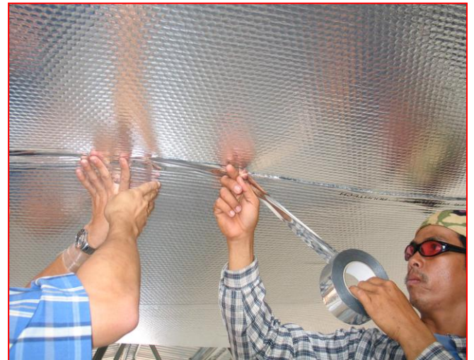
Once Polynum is attached, tape is used to seal over laps
