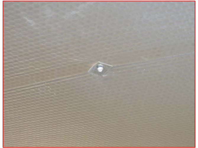
Screw and washer used to attach Polynum to metal frame
