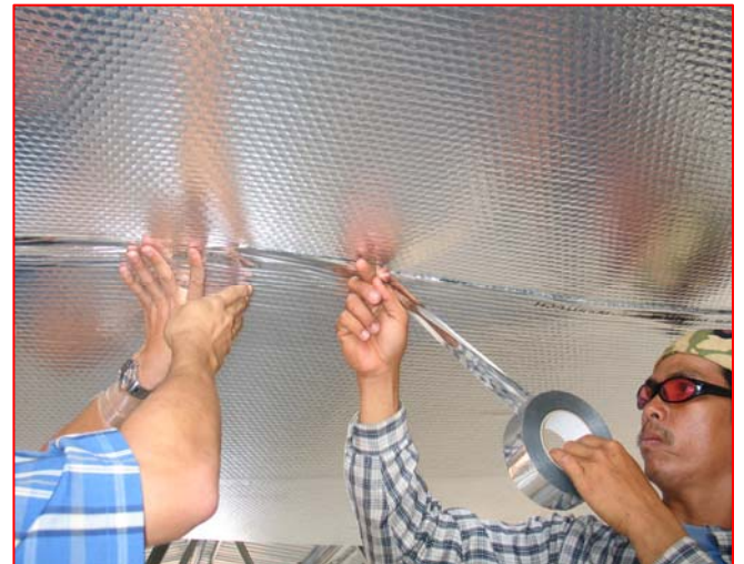
Once Polynum is attached, tape is used to seal over laps
