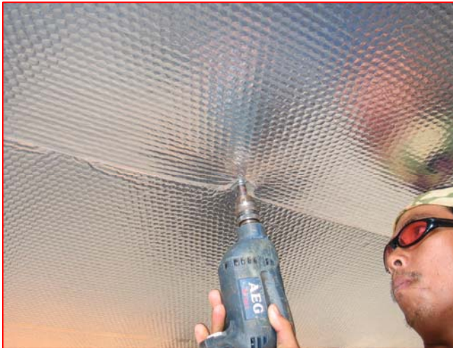
Self-tapping screws are used with wide flat washers
