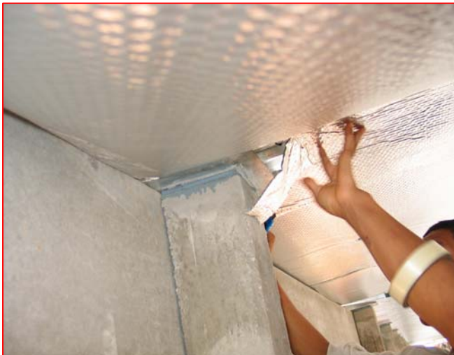
Cutting and aligning the edges
